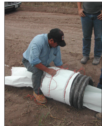
Figure 5c. Making a tight connection to avoid water leaks.
