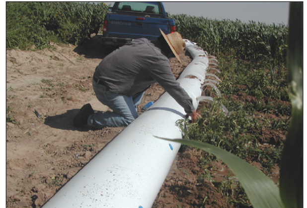
Figure 8a. Inserting plugs in poly-pipe.
